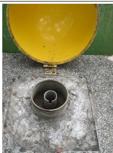
量測導管俯視
