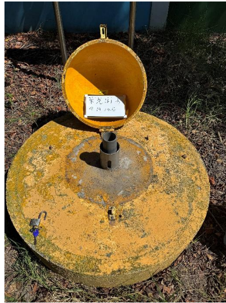
量測導管俯視
