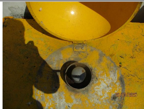
量測導管俯視
